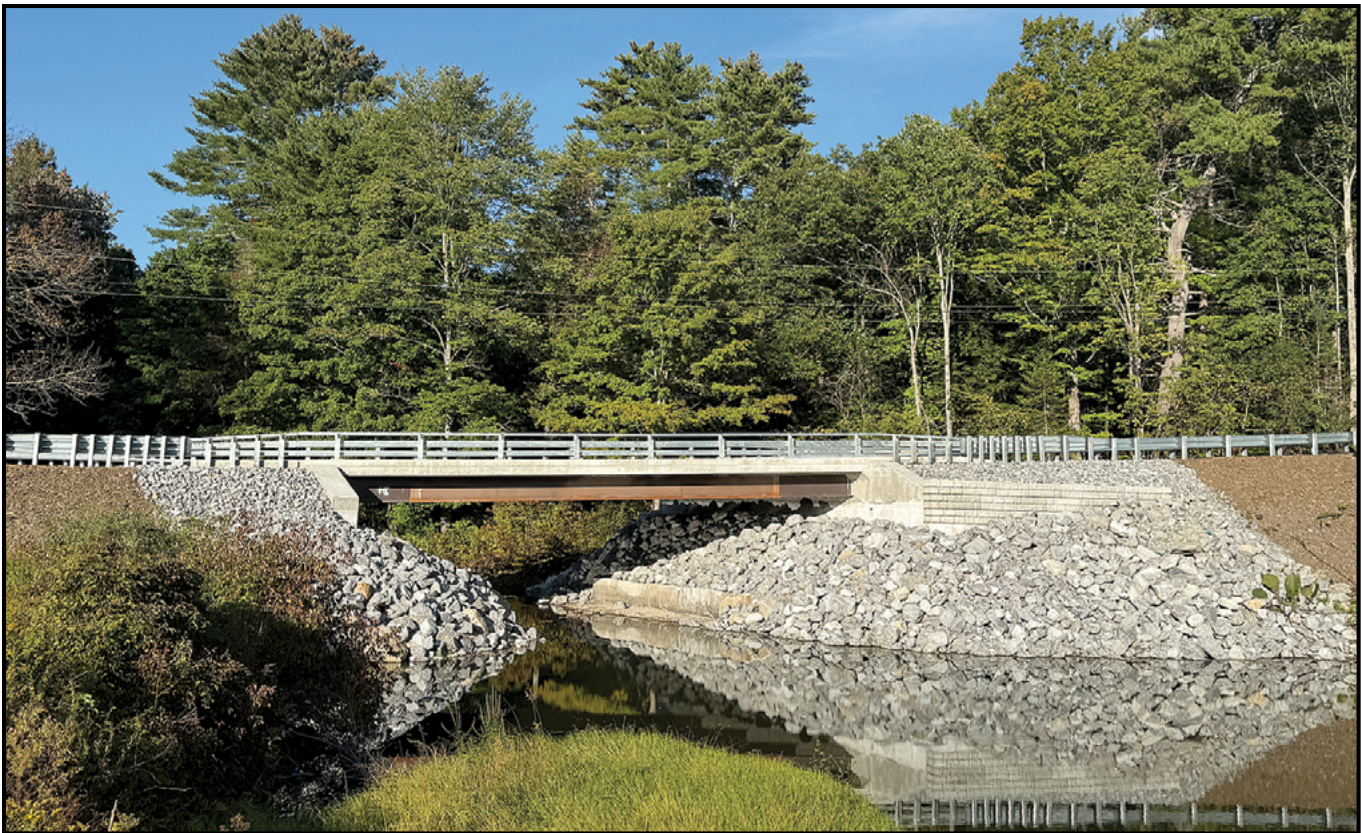
Construction to replace Varney's Bridge on William Knight Road over the Pleasant River in Windham has been completed three weeks ahead of schedule and the bridge has been reopened. Work to demolish and replace the aging 26-foot steel girder bridge began there on June 15. PHOTO BY KEITH MANK
