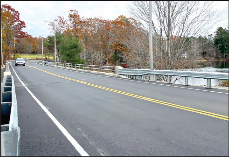
After being closed for 53 days, the Great Falls Bridges linking Windham to Gorham have reopened to the public. The project cost almost $400,000 and work was intended to improve the condition of the existing bridge structures while preserving the existing deck and superstructure longevity of the bridges. PHOTO BY ED PIERCE
