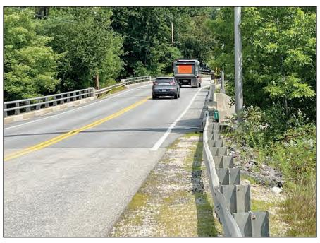
Crews will start work on the Great Falls Bridge connecting Windham and Gorham on Aug. 18. The project involves 350 feet of approach work, replacing guardrail transitions and flare terminals, and expansion joint modification. A light pole will also be removed. PHOTO BY ED PIERCE
