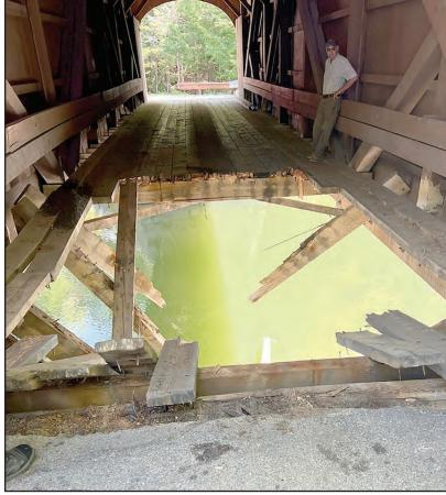
Babb's Bridge, a wooden covered bridge over the Presumpscot River, will be closed until at least next spring after a truck weighing six times over the 3-ton limit attempted to cross limit of 10 feet and the from Gorham into Windham on Aug. 23 and crashed through bridge is covered by a the bridge floor. PHOTO BY GORHAM POLICE DEPARTMENT
